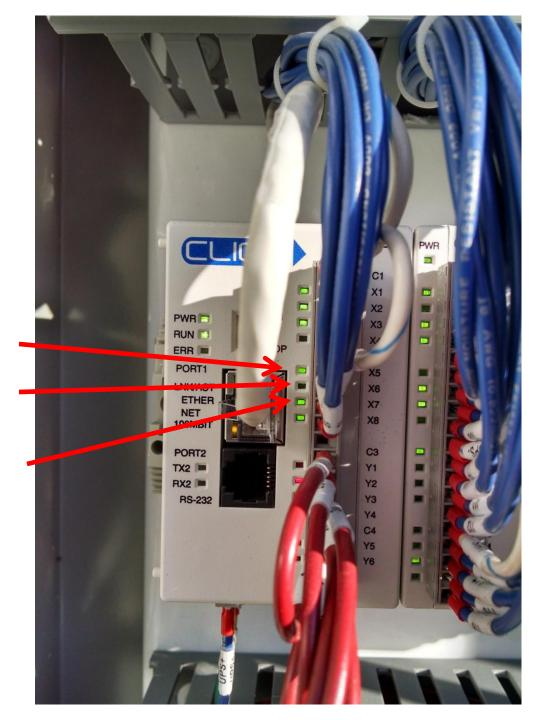
The easiest way to test the floats is to remove the floats from the sight tube. With the float tree in the upright position, all of the floats will be in their resting position. Look at the PLC and note the status of the input lights. In this AWS example the lights will be off, off, on.
